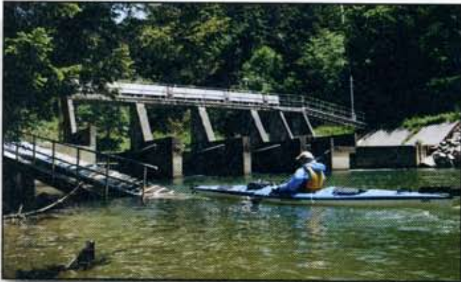
A portage about halfway between the lake and the ocean helps paddlers get around a small dam.
